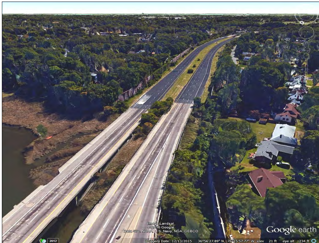
Figure 2-4: I-64 in Norfolk (Looking South)
