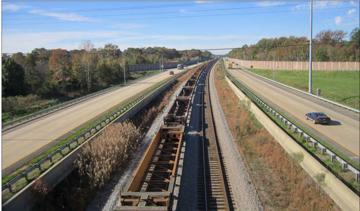
Figure 2-5: VA 164 Looking West
