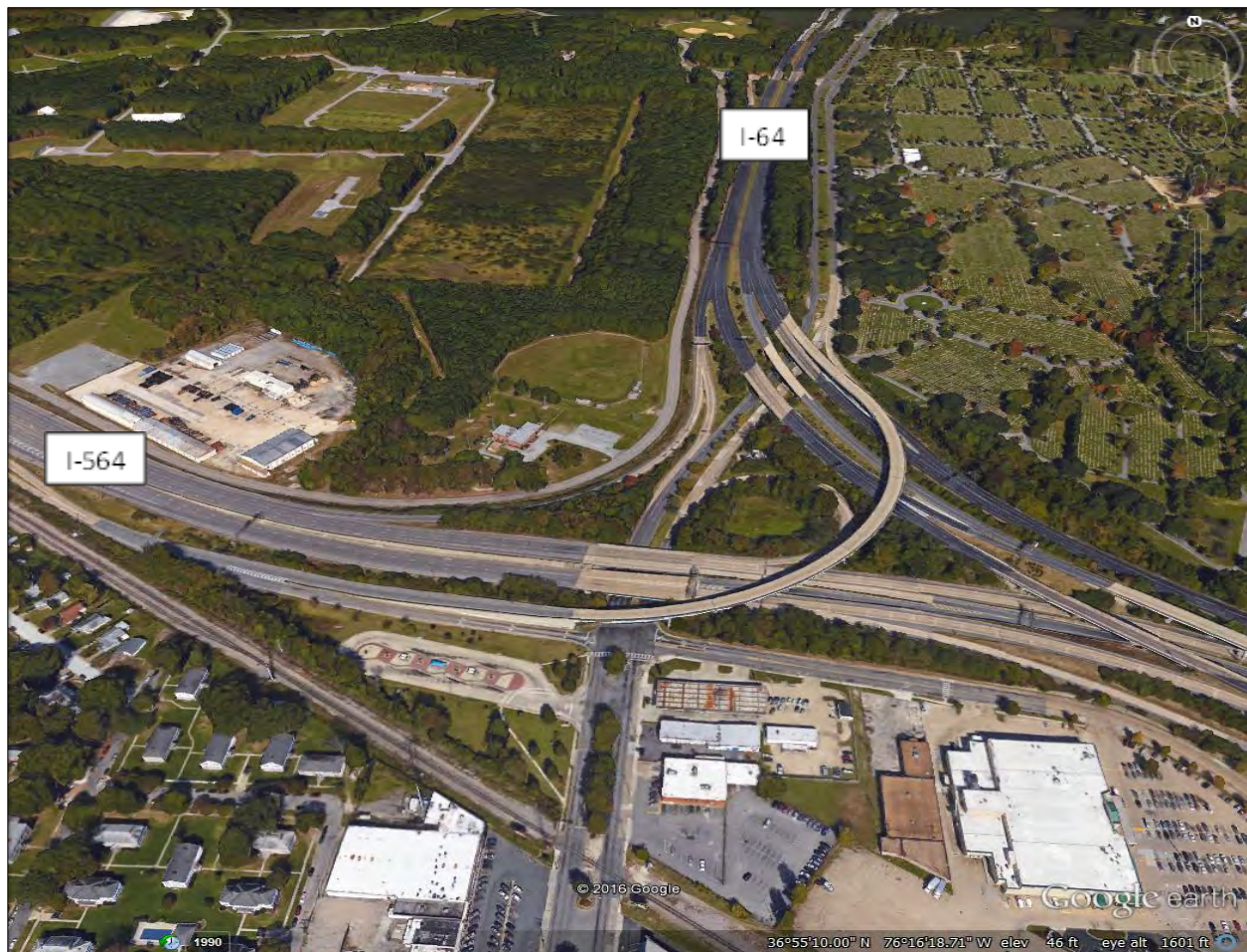
Figure 2-6: I-64/I-564 Interchange (Looking North)
