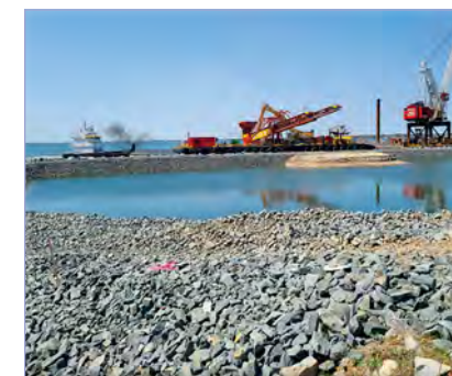
The sand fill process has started on the North Island.
