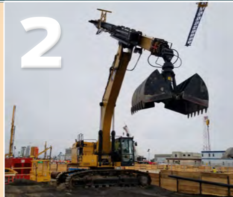
1 Aerial view of the South Island. 2 A teledipper removes excavated soil from the launch pit. 3 A view of the launch pit where crews are preparing the headwall. 4 A crane lowers the sealing ring, which serves as an interface between the TBM and the tunnel approach structures. 5 An aerial view of the TBM launch pit. 6 Crews install the base slab at the bottom of the launch pit.
