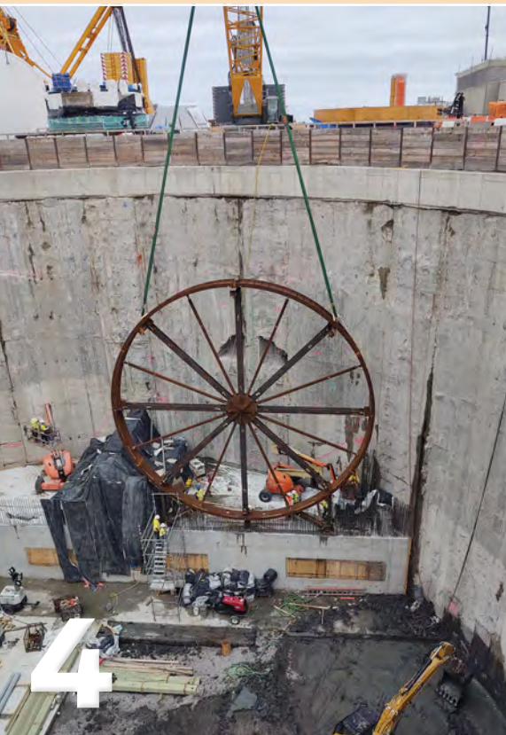
1 Aerial view of the South Island. 2 A teledipper removes excavated soil from the launch pit. 3 A view of the launch pit where crews are preparing the headwall. 4 A crane lowers the sealing ring, which serves as an interface between the TBM and the tunnel approach structures. 5 An aerial view of the TBM launch pit. 6 Crews install the base slab at the bottom of the launch pit.
