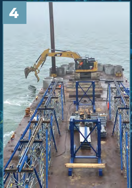
[CLOCKWISE]: 1 A map shows the locations of the VMRC artificial reefs. 2 3 4 Placement of 70 tons of concrete material at the Back River Reef.
