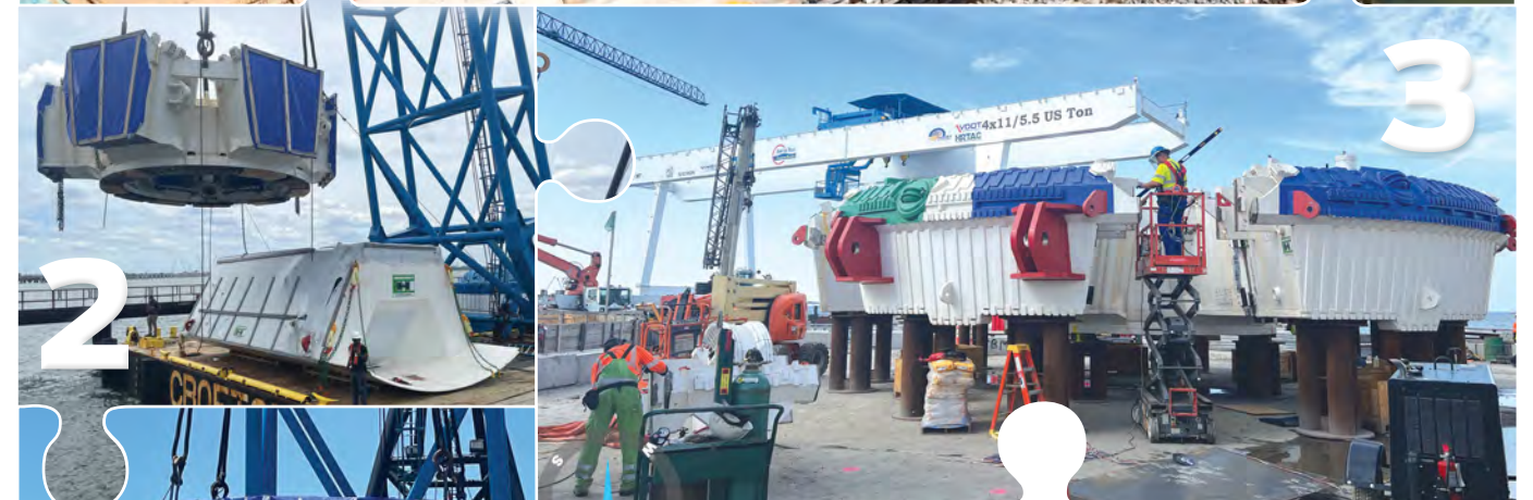
1 An aerial view of the assembled tailskin. 2 Pieces of the shield are moved from the barge to the island. 3 Crews assemble the cutterhead. 4 A crane lifts the main drive. 5 Inside view of crews welding together the tailskin.
