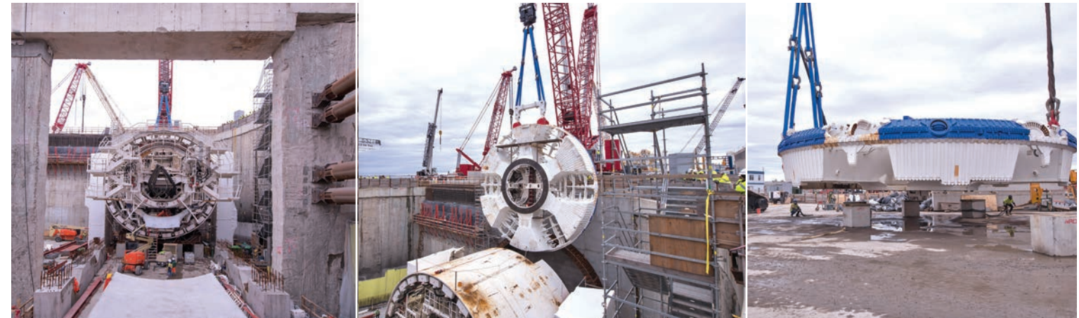
[LEFT TO RIGHT]: 2 A view of the TBM shield from the first trailing gantry. 3 The TBM cutterhead is lowered into place. 4 Cranes lift the TBM cutterhead so crews can remove the concrete support blocks. 5 The crane swings the TBM cutterhead into position over the launch pit. 6 VDOT Project Director Jim Utterback and HRCP Project Manager Louis Brais take a minute to celebrate the progress.
