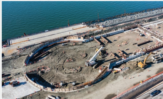
Crews prepare to begin excavation of the TBM receiving pit.
