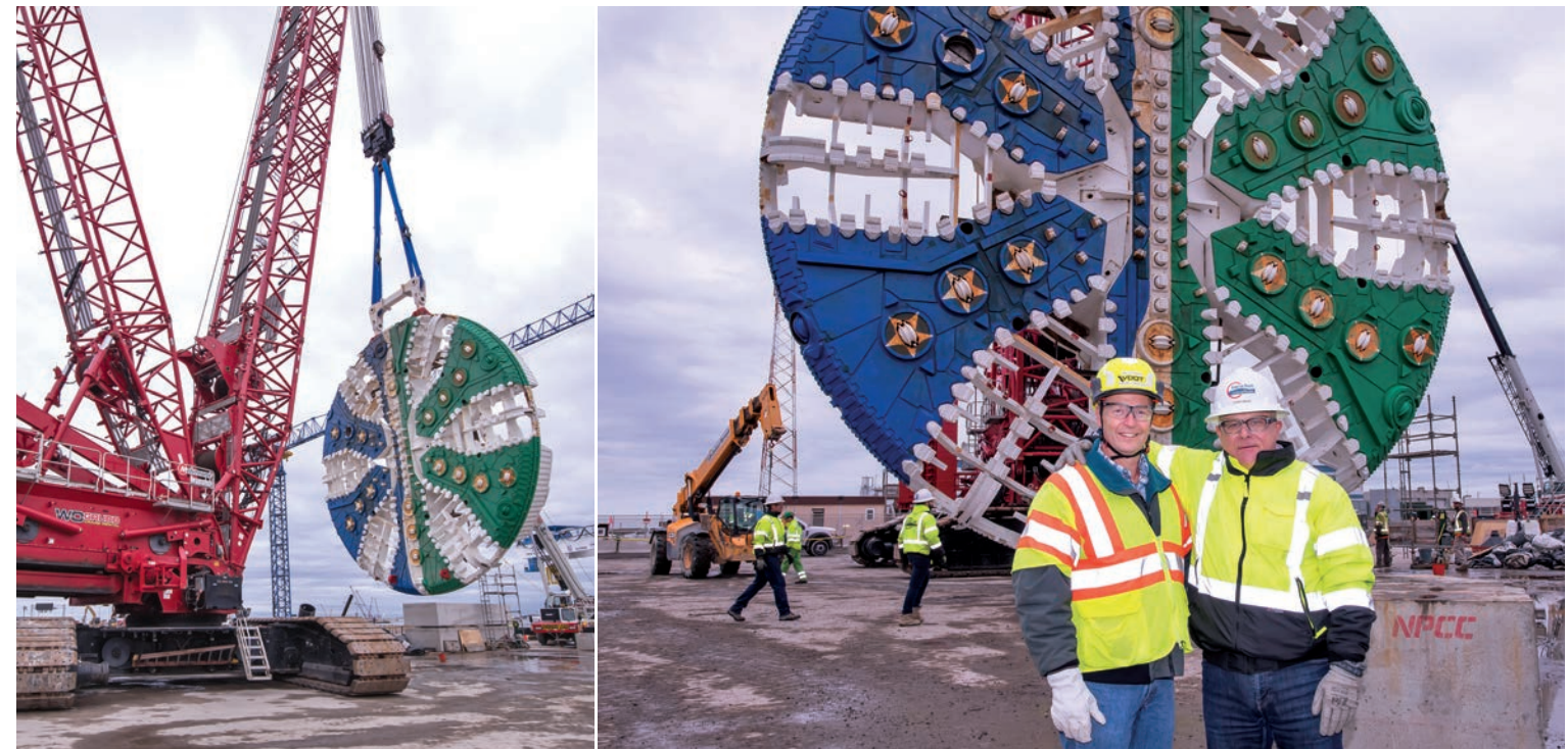
[LEFT TO RIGHT]: 2 A view of the TBM shield from the first trailing gantry. 3 The TBM cutterhead is lowered into place. 4 Cranes lift the TBM cutterhead so crews can remove the concrete support blocks. 5 The crane swings the TBM cutterhead into position over the launch pit. 6 VDOT Project Director Jim Utterback and HRCP Project Manager Louis Brais take a minute to celebrate the progress.
