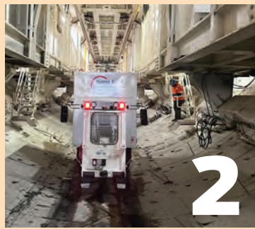
[ABOVE]: 1 The TBM operator monitors all operations from the control room. 2 Multi-service vehicles are used to transport the tunnel segments to the TBM. 3 The segment feeder brings in tunnel segments as the vacuum erector awaits overhead, preparing to move each segment into place. 4 The TBM has 54 hydraulic thrust cylinders that push against the tunnel ring to move the TBM forward.
